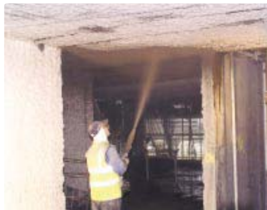
Figure 7: Application of sprayed concrete to repair a fire-damaged slab soffit following removal of fire-damaged concrete.
