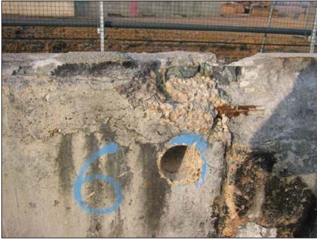
Figure 4. Main bund joint (with core sample 6 cut through it)
