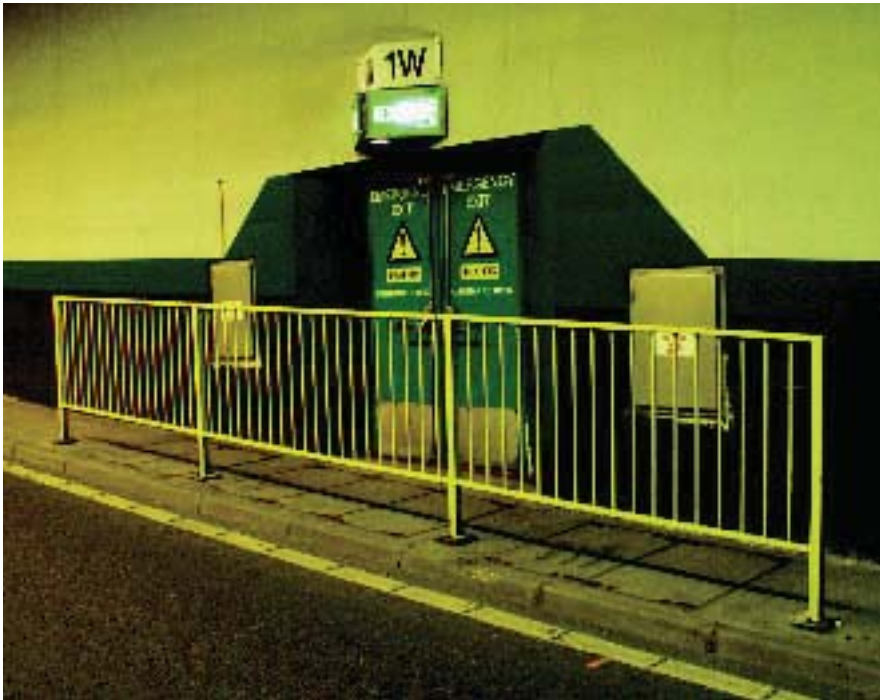
Emergency exit at Medway Tunnel
