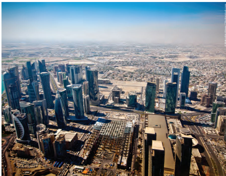
Doha, the capital of Qatar, will soon have a metro network and heat exhaustion was a key design issue for the ventilation and cooling of its four lines
