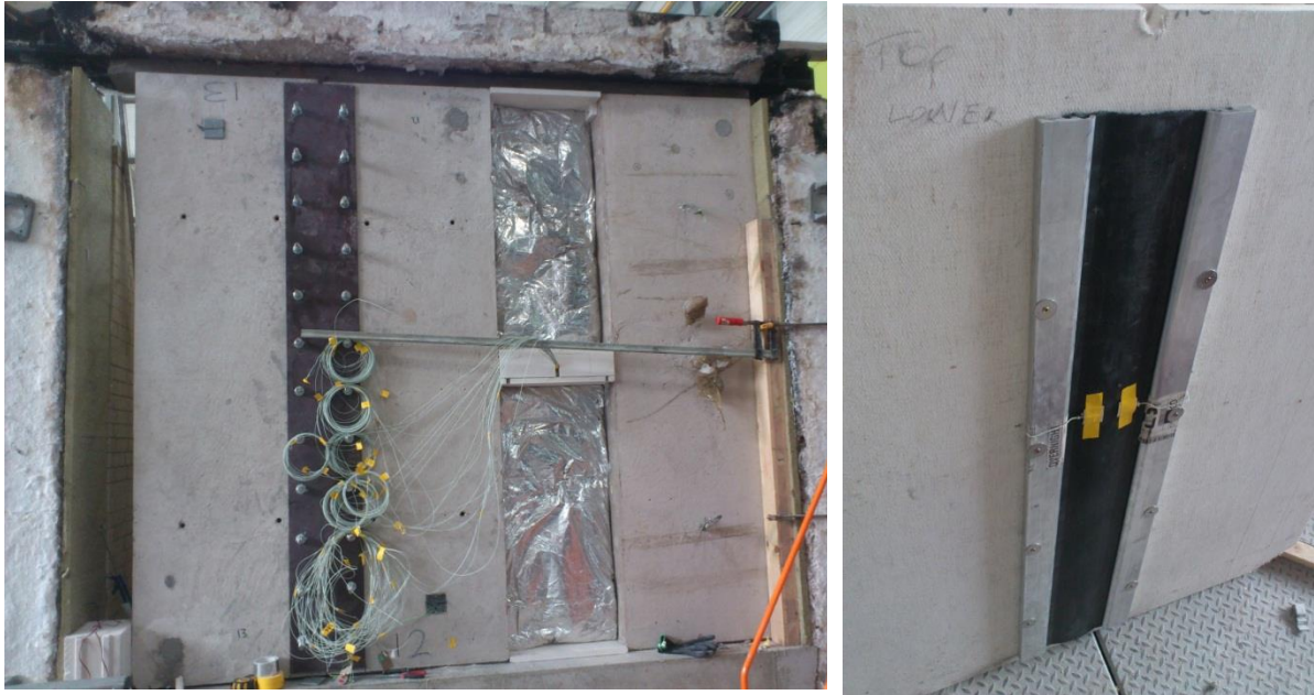
Figure 7: Vertical (Wall) Element Fire Test: Preparation of the insulation material and thermocouples positioned on the joint ('cold' side)
