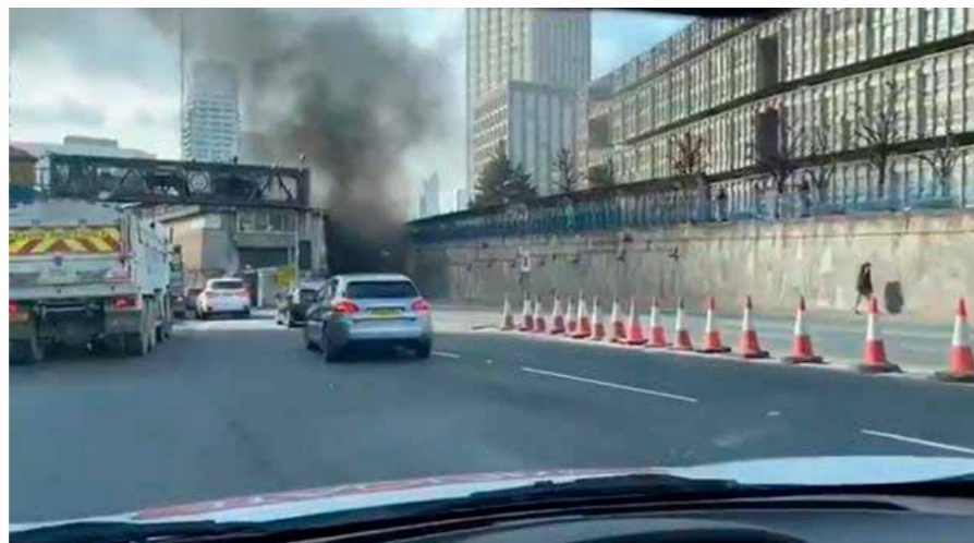
▼ Smoke billowing out from the Blackwall Tunnel.
