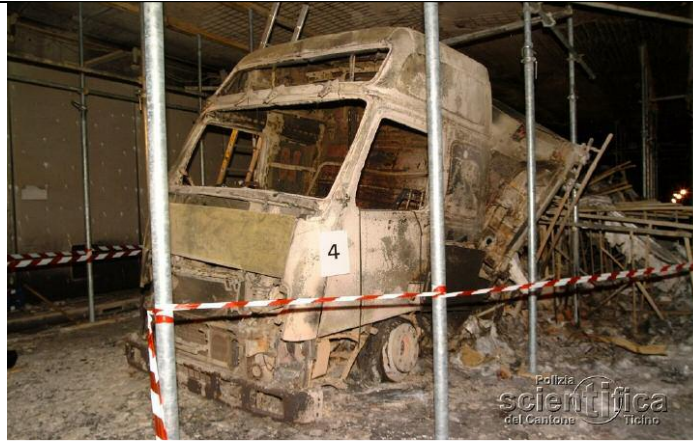
Figure 1: Support of the suspended ceiling at risk of collapse.
