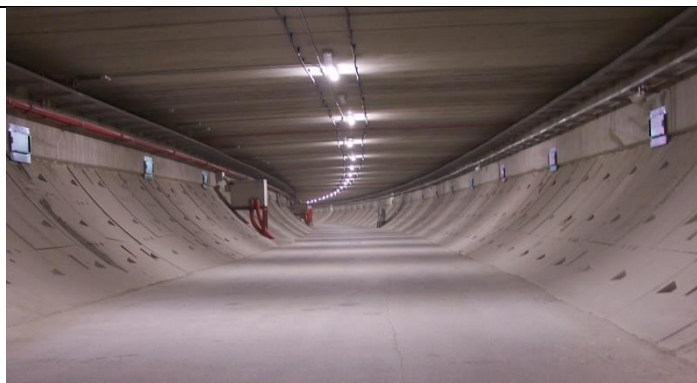
Figure 7: Emergency Gallery under road level from South By Pass Tunnel.
