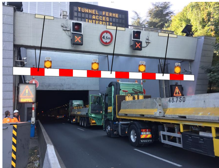
Figure 2. Arrival of the reinforced concrete barriers to protect the shoring
