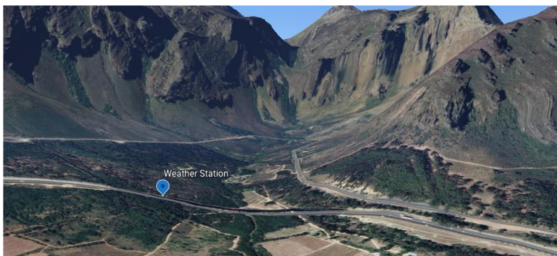
Figure 3 – Setting of the Hugo River Viaduct
