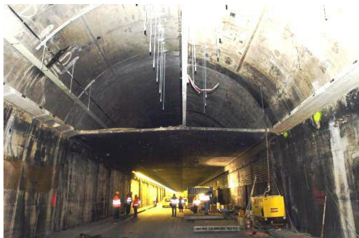
Figure 2: Situation before assembly of the ceiling elements.
