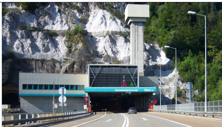
Figure 2: Northern Portal of the Karavanke Road Tunnel
