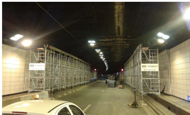
Figure 3. Shoring and metal beams to stabilize the vault
