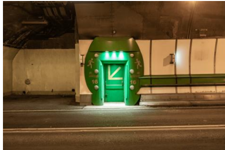
Fig. 12. Post-Fire emergency escape routes
